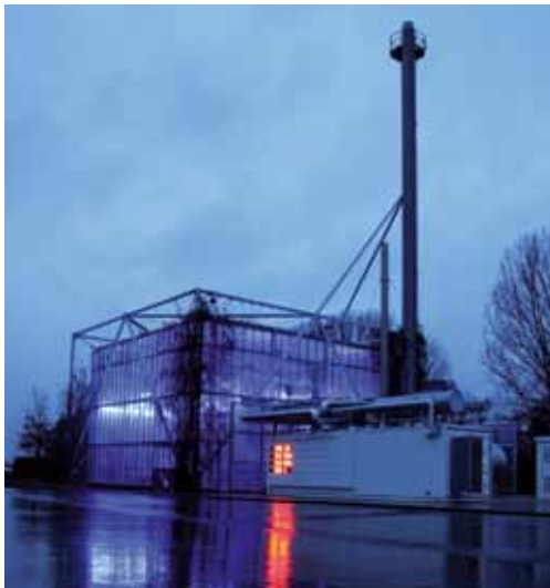
Co-generator powered by renewable raw materials
